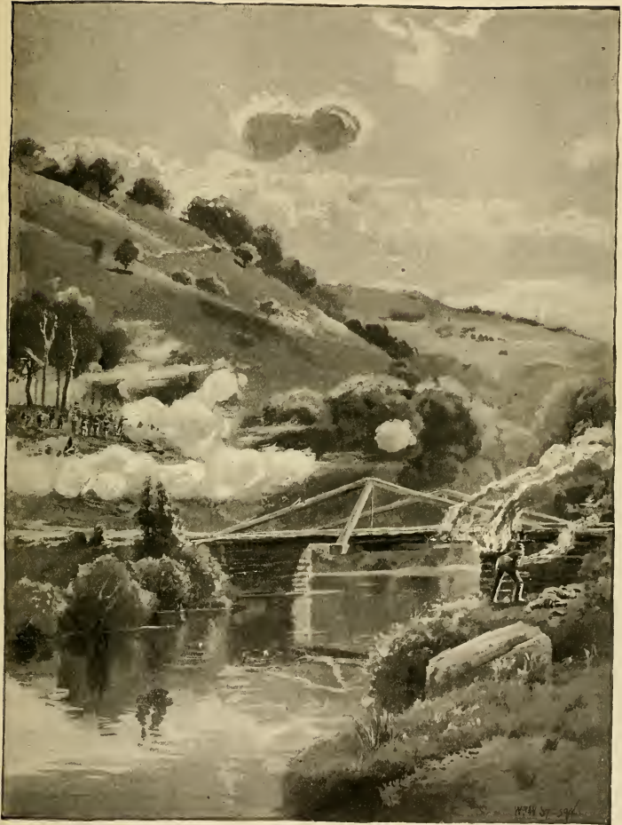
DESTROYING THE BRIDGE AT FRONT ROYAL, VA.
